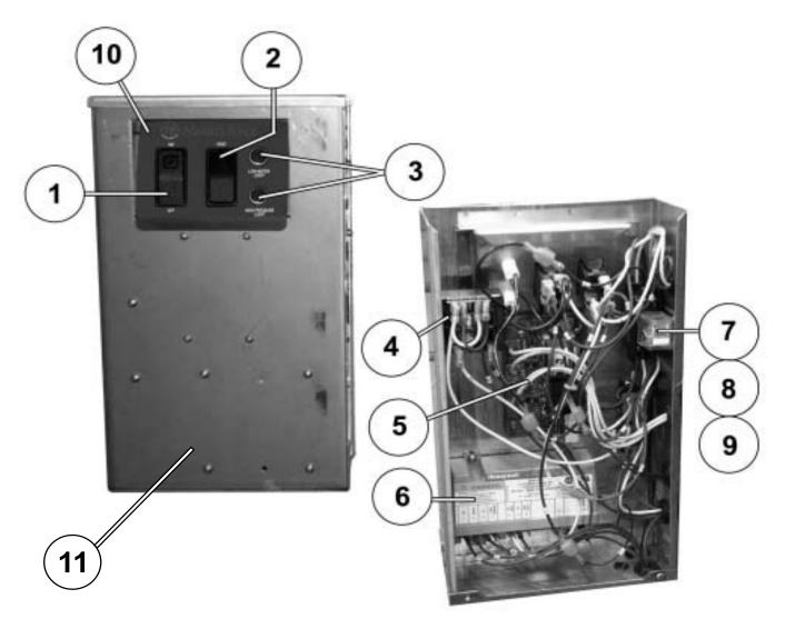
Control Box Assembly, with and without Cover
